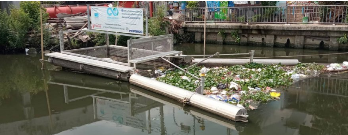
Trash trap in the Lat Phrao Canal in Bangkok, Thailand operated by TerraCycle Thai Foundation. Credit: TerraCycle Global Foundation
